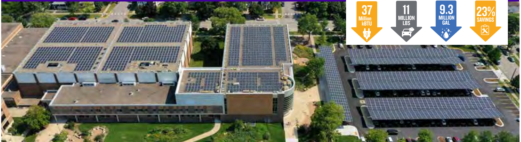
Completed Energy Savings Project Phase 1 (Spring 2023). (FPG 10)
